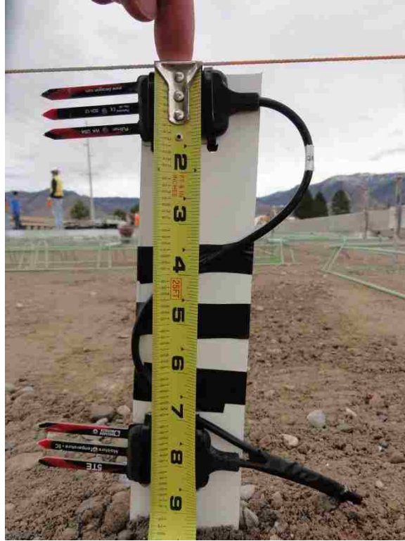
Figure 3-4: Temperature and moisture sensors for monitoring concrete pavement.
