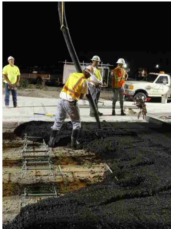
Figure 3-7: Placement of darkened concrete.
