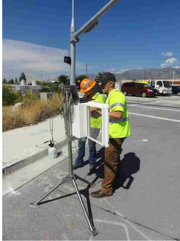
Figure 3-9: Measurement of pavement albedo.
